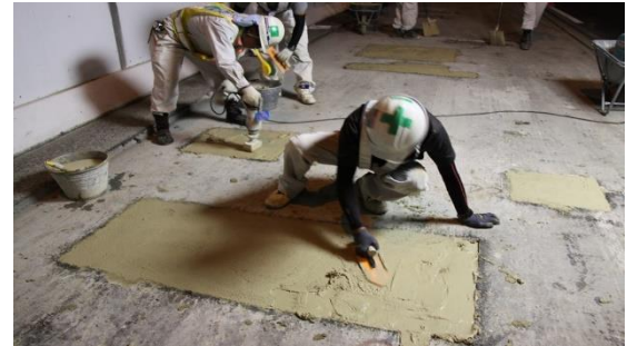
Patching by Repair mortar
