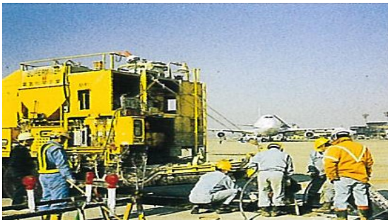
Repairing for apron of Airport
