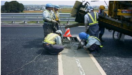
Repairing for expansion joint of Bridge
