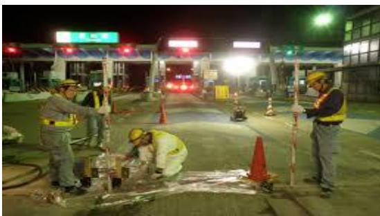
Repairing for Tollgate of Highway
