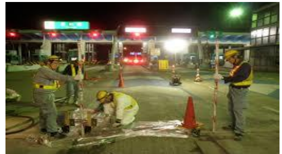
Repairing for tollgate of high way
