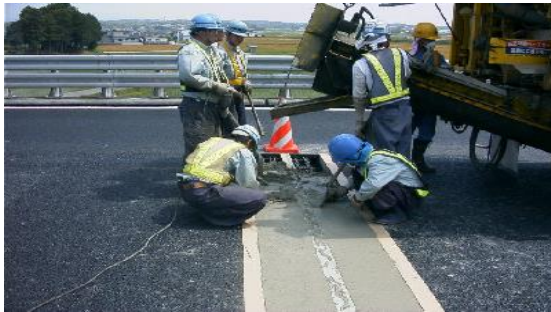
Repairing for expansion joint of Bridge
