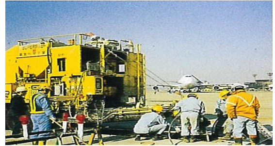
Repairing for apron of Airport
