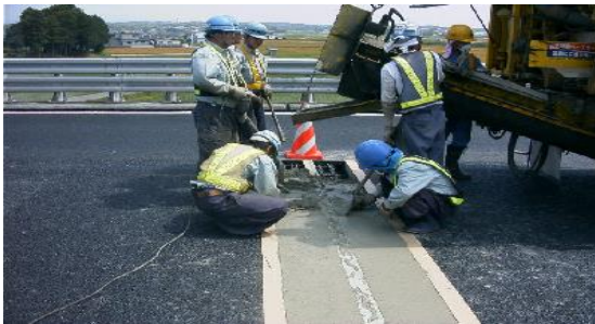
Repairing for expansion joint of Bridge
