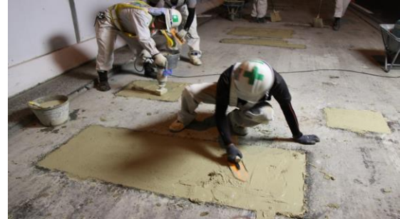
Patching by Repair Concrete
