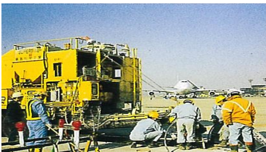
Repairing for apron of Airport
