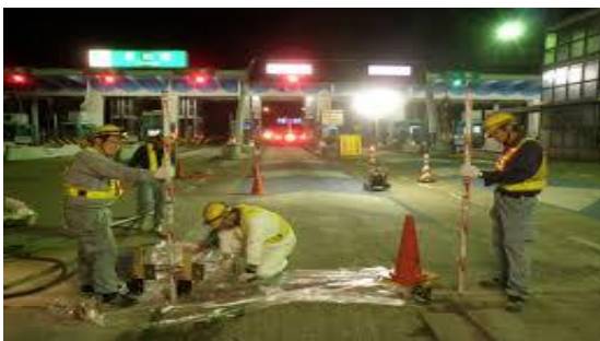
Repairing for Tollgate of Highway
