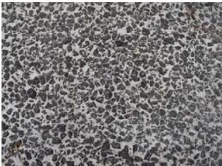
Semi-rigid pavement with asphalt
