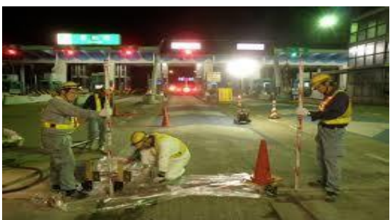
Repairing for Tollgate of Highway
