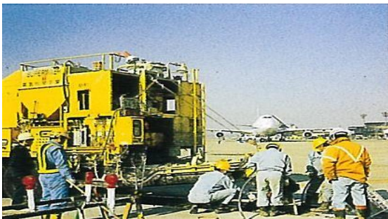
Repairing for apron of Airport
