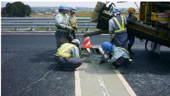
Repairing for expansion joint of Bridge
