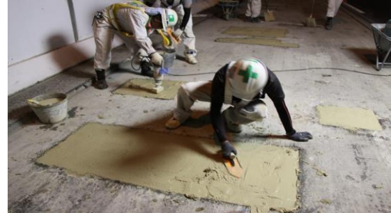
Patching by Repair Concrete
