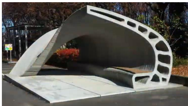
Shell-shaped bench built up by 3D printing
